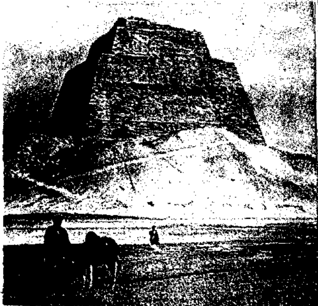
AT MEDUM, on the desert's edge, forty miles south of Cairo, is the queerly shaped pyramid of King Sneferu. It rises in three tiers from a mound that is really another tier covered with debris. Most likely it was once a true pyramid in shape. King Sneferu built for himself another pyramid at Dashur, but it was probably in this one that he was buried.
